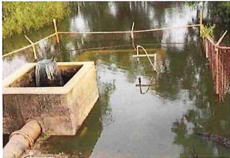
Picture 1 was taken on March 10, 2023 and it shows the flood waters starting to rise around the chlorine contact chamber and weir box at the existing wastewater treatment plant.
