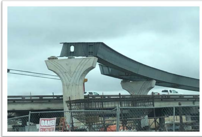
Steel Tub Girder Erection
